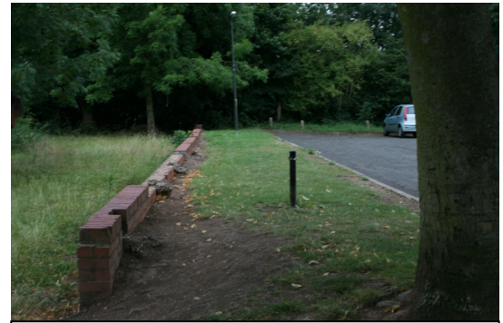
Perimeter wall along Swanslength
